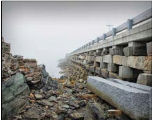
Photograph, The Cribstone Bridge. Howard Search
