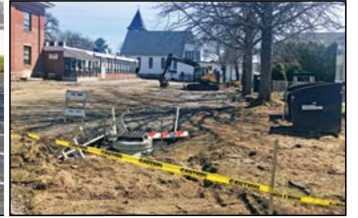
AWAITING MEMBERS ARRIVAL back at People Plus is a brand-new parking lot with all the trimmings. According to Ryan Barnes, Town Engineer of Brunswick, the newly completed project includes the replacement of the existing paved surface, installation of a closed-drainage system, and a new raised sidewalk adjacent to the building. Also, the existing pavement between the trees along the edge of the parking lot was removed and replaced with loam and seed to help protect the trees in the future. The People Plus parking lot was last constructed nearly 20 years ago.
